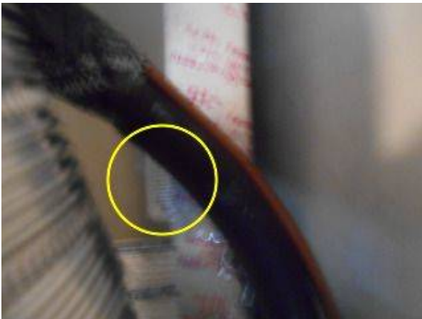
Photo 3-1 air handler label covered
