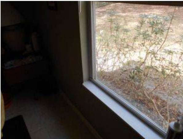
Photo X-5 Al dbl pane SH windows excellent condition
