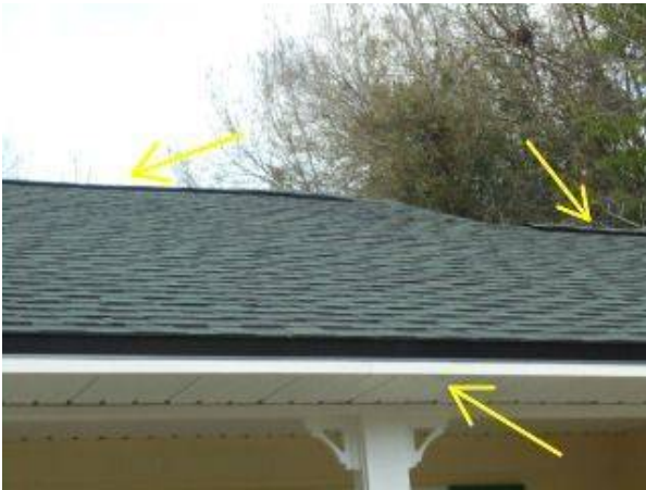
Photo X-9 New roof 3/12 pitch arch shingles ridge/soffit venting excellent
