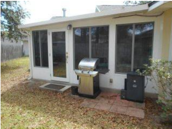
Photo X-11 sun room / hot tub area no issues observed
