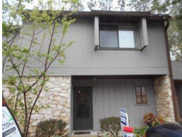
Photo 14-2 well maintained grounds, exterior doors and windows sealed and maintained well.
