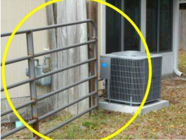
Photo 2-1 proximity of gas meter and AC
