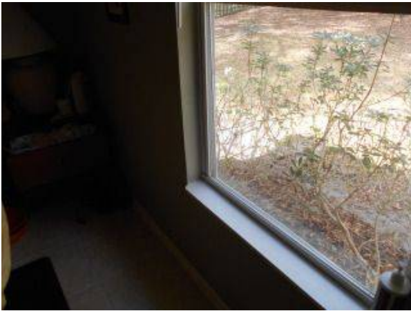
Photo X-5 Al dbl pane SH windows excellent condition
